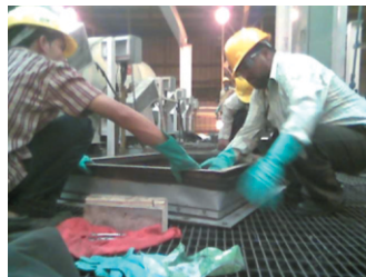
Installation of Fabric Comapanensators at site
